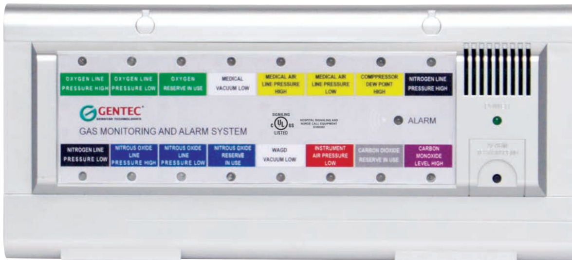
GUMACSTM Series Master Alarm (up to 32 inputs)
